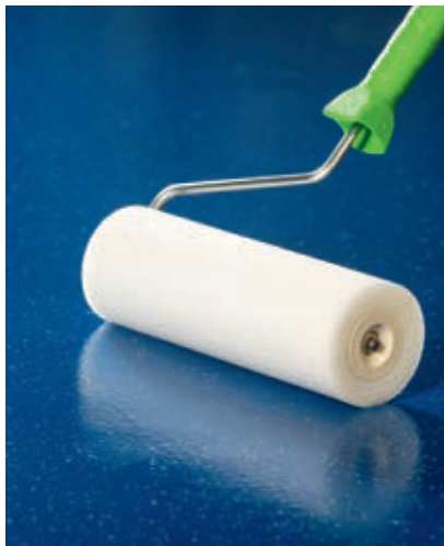
Sealing after strewing with chips
